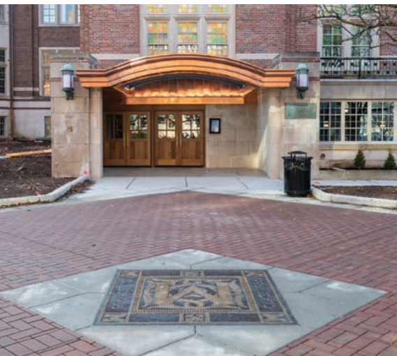
A canopied entrance on the north side of the building includes an ADA-accessible ramp, just one of the many building changes designed to increase access.
